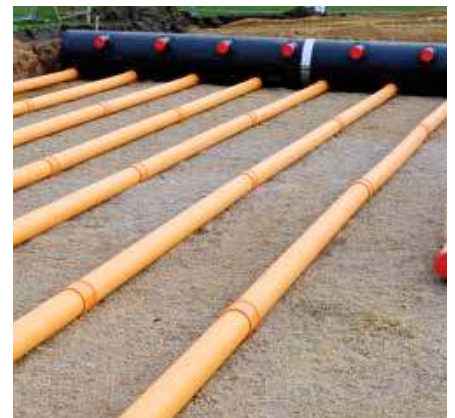
Ground-air heat exchanger
