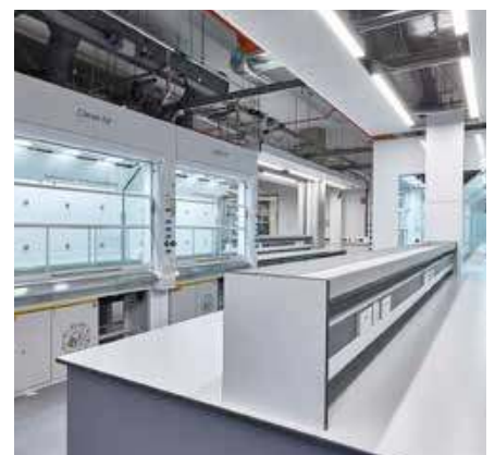
Innovative uses of cable trunking
